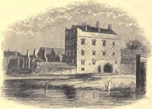
THE GATEWAY, CROYDON PALACE.
